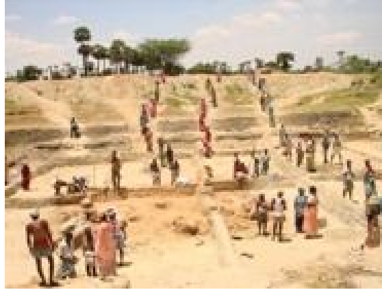
Desilting of Pond
